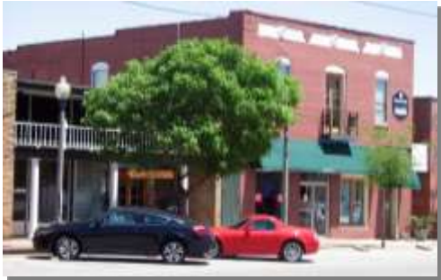
Figure 8.10: Shops along Hoyle Ave. South
