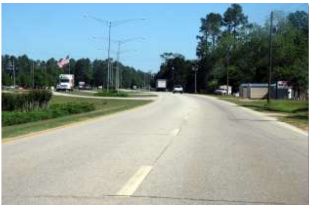
Figure 4.8: HWY 59/31 south, northward bound approaching Bay Minette City limits
