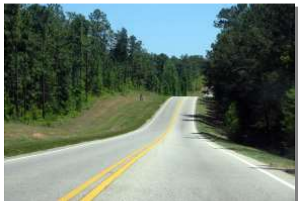
Figure 4.3: HWY 59 north of Bay Minette, southward bound
