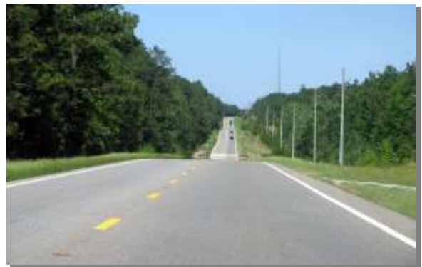
Figure 4.16: HWY 31, eastward bound to Escambia County
