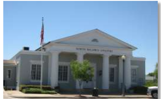
Figure 9.9: North Baldwin Utilities
