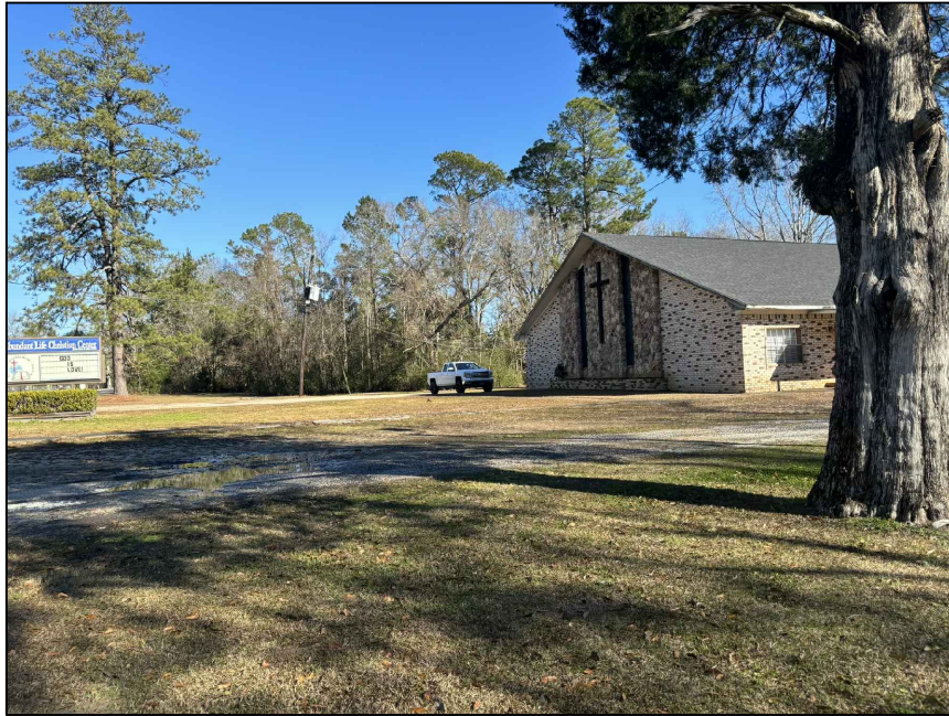
General view of the church onsite.
