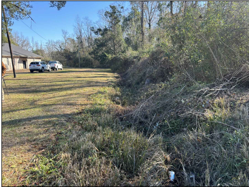
General view of D-1 located in the southwest corner of the site, extending east.
