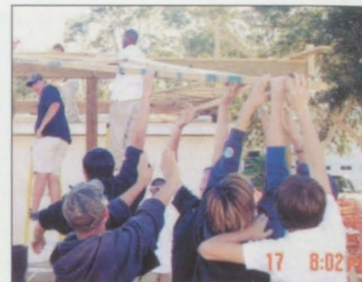
Right: Hold it up... The Building Construction class is helping hold up the unfinished roof.
