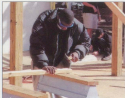
Left: Working hard... William Anderson is hammering away.
