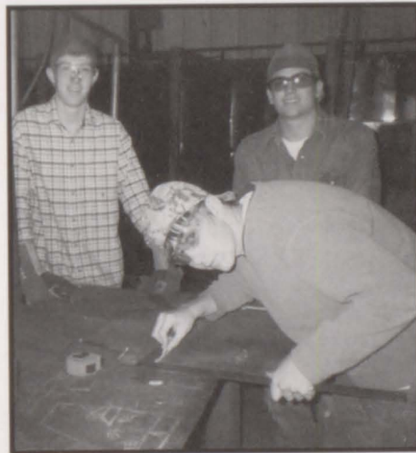
Kaston Peavy, Nich Scarbrough, Clay Shiver layout and mark the armor door panels for the National Guard humvee project.
