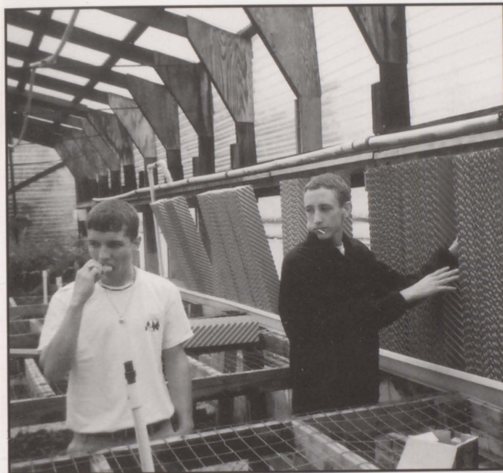
John Black and Kevin Johnson learn how to install panels for the new cooling system.
