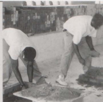
Left: A race to the finish... Jarrod Jennison and Bernard Johnson work on building brick corners for class.
