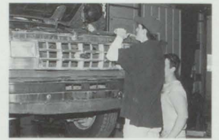
Open Hood... Mickey Brooks and Daniel Smith bleed the clutch.
