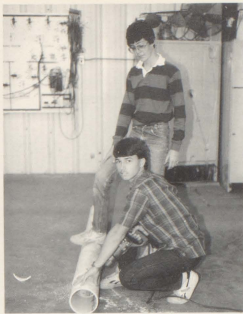
Gayland Hadley and Barton Phillips are cutting on PVC pipe.
