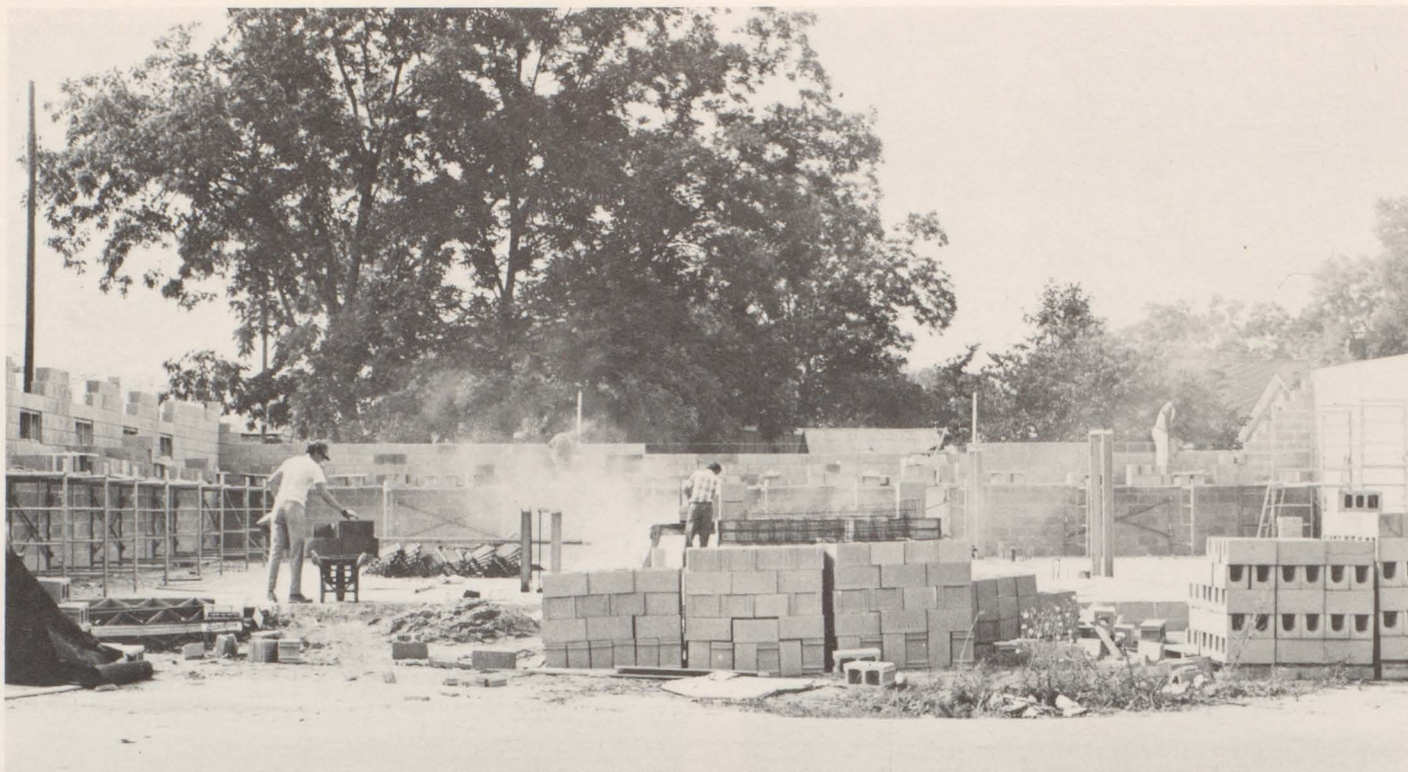
Stuart Construction Company helps build Bay Minette.
