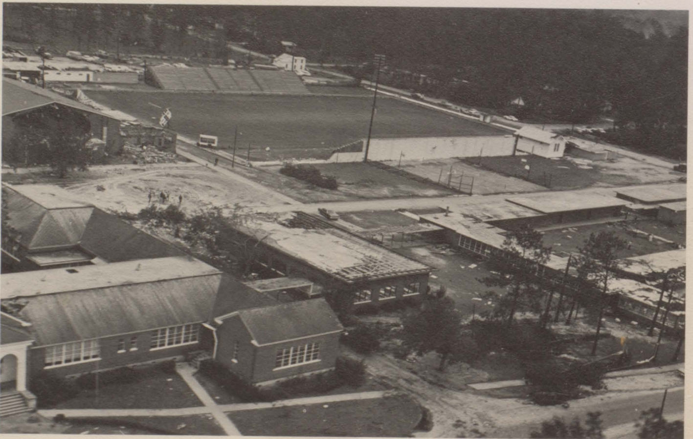
Damage to BCHS, as seen from the air, is extensive.
